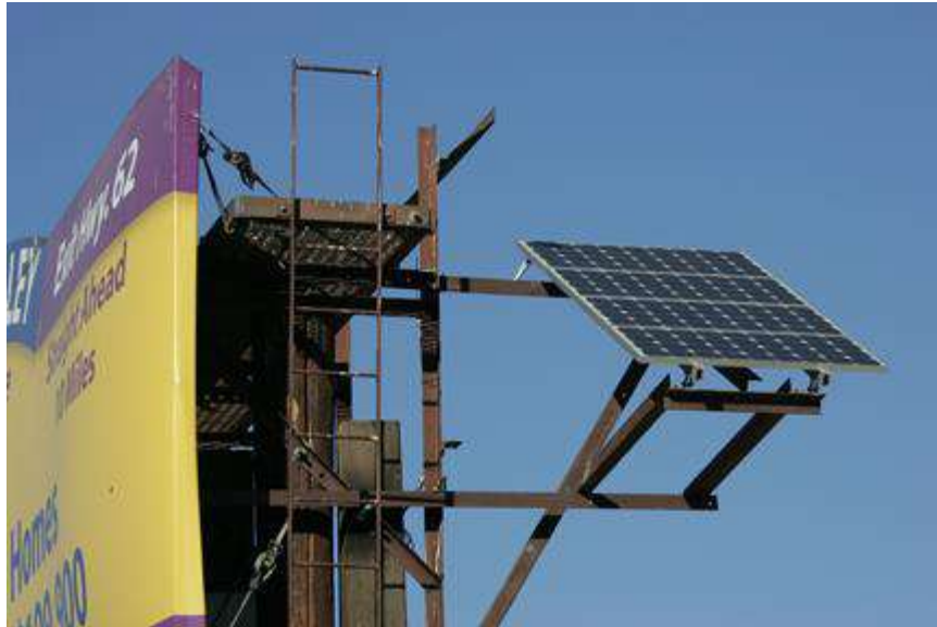
Figure-1: Solar powered light for Hoarding
