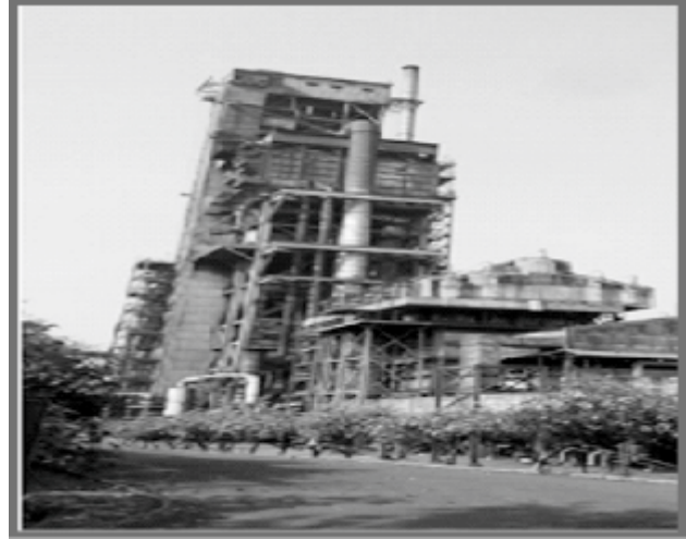
JSW Steel Plant
