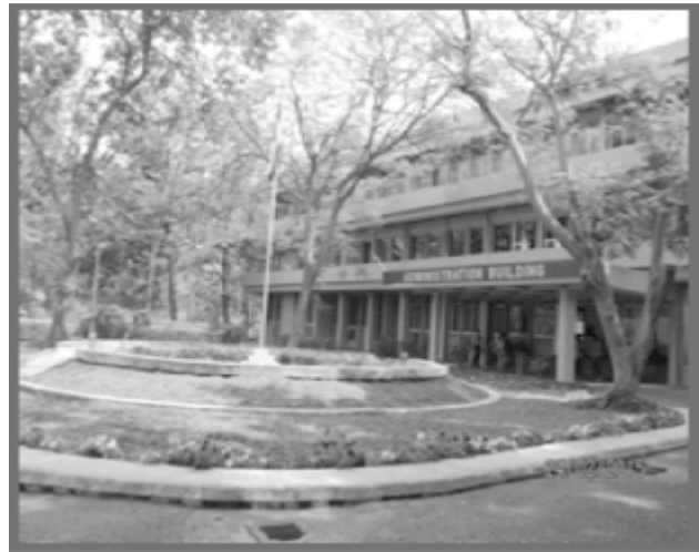
JSW Steel Plant
