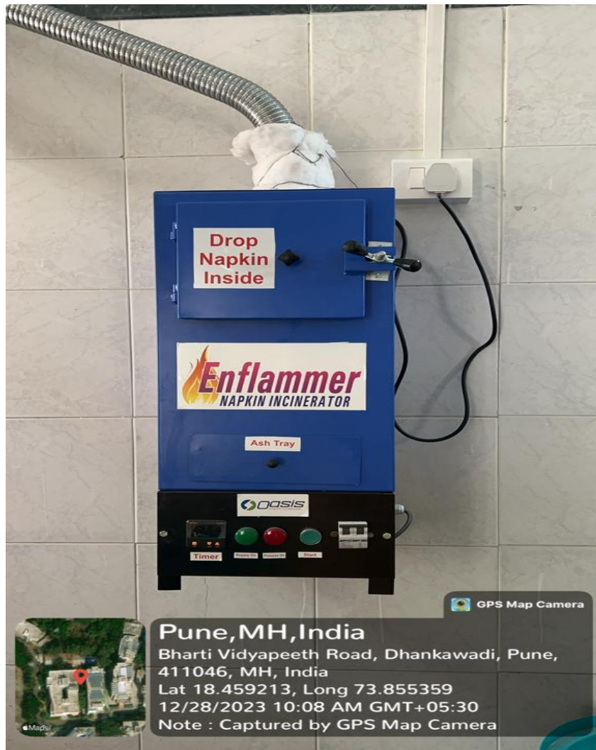
Sanitary Napkin Incinerator
